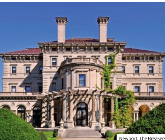
Newport, The Breakers
